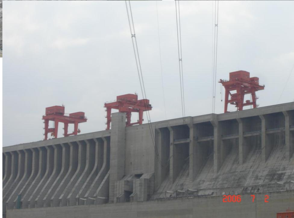
Large pulley machines to control flow of water.
