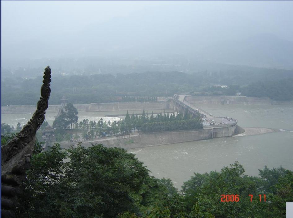
The Dujiangyan Irrigation System diverts water from the Minjiang River (a tributary of the Yangtze), supplying Chengdu with fresh water and preventing floods.
