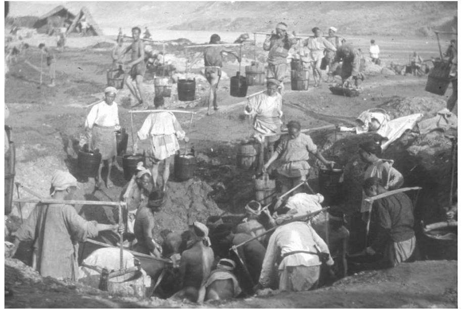
Workers collecting salt water from surface springs at Kweifu (Fengjie). The water is boiled away in vats.
