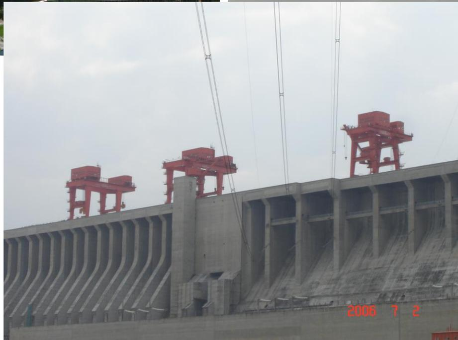
The pulley machines that lift the large metal spillway doors
